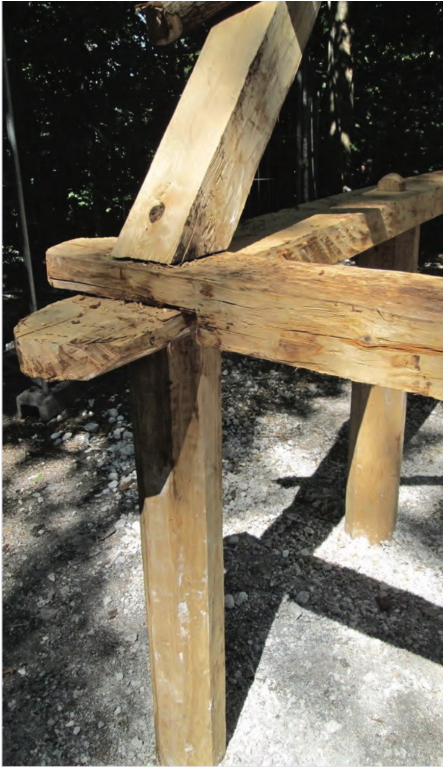
Details of the corner of the building showing dowels.
